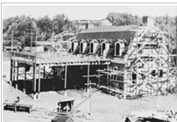
The Sumas Border Inspection Station Under Construction in 1932.
